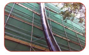
Wear resistant plastic chutes, quiet in use and easy to transport and erect. Fixings
