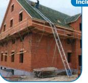
Will lift up to 200kg; an extending scaffold bracket makes it possible to handle bulky loads. Lifting heights of 25m or 50m at 30m/min are safely achieved using a non-twist 5mm wire rope. The pendant control includes an emergency stop button and the bracket swivels for safe loading. Can be used free-standing, with a cantilever frame,
