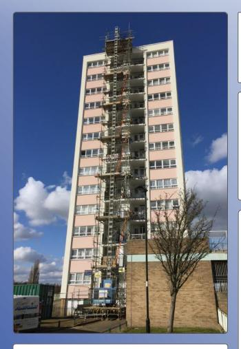
This double barrow rack and pinion hoist can be used for materials only. The "Double Barrow" hoist's cage is twice the size of the regular Geda 300Z's, so is ideal for more bulky loads up to 300kg - Geda 300Z Double Barrow hoists can be attached to scaffold or directly to a building using wall mounts.
